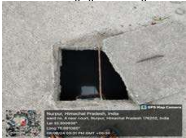
Rain water harvesting
